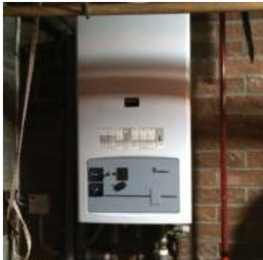
Before and after the installation. The box-off, box-on solution minimises disruption and redecoration.
